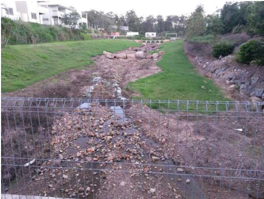
Figure 3 – Reinstatement of local drainage path
