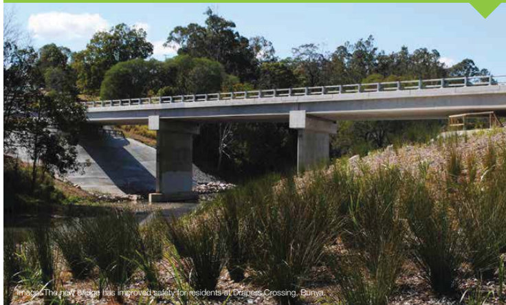
Image: The new bridge has improved safety for residents at Drapers Crossing, Bunya.
