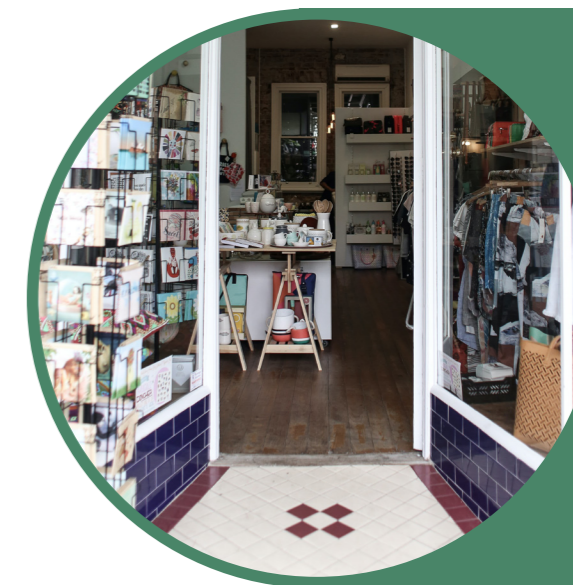
Ramped doorways, set back from the property line, allow more people to access your business than stepped doorways.
