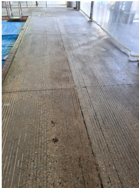
Figure 5: Image of Expansion Joints
