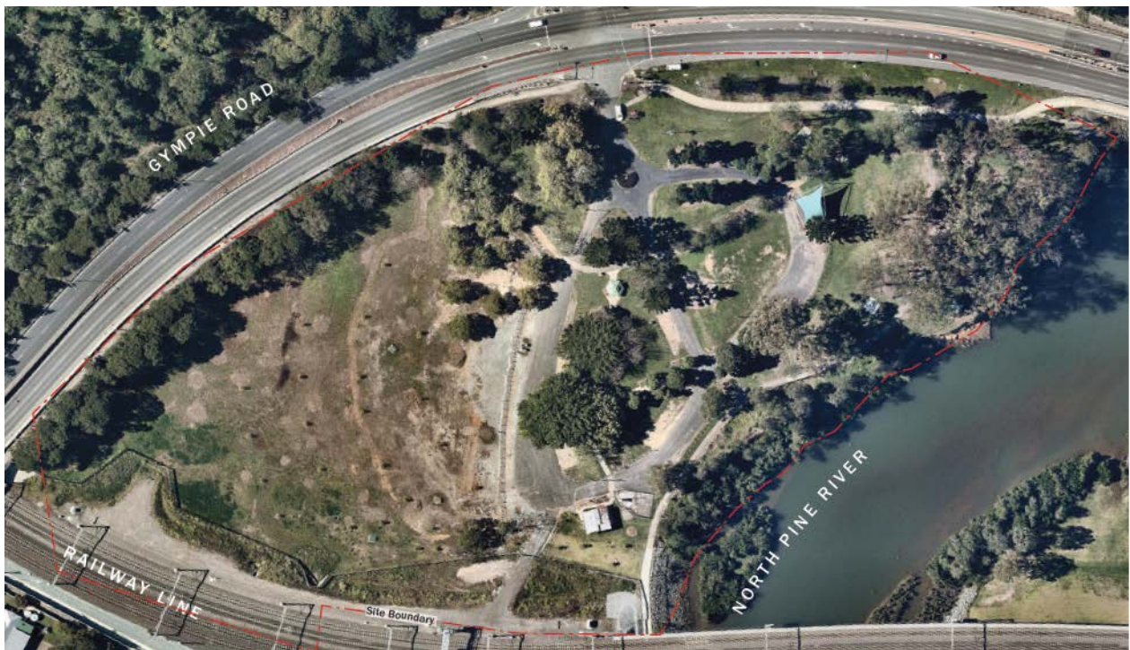
Figure 4: Wyllie Park Aerial Photo, 2017 showing the programmed replacement of trees triggered in part by the MBRL rail corridor expansion
