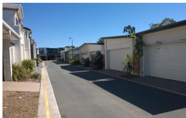
Laneway Houses (Front and Rear) (Fitzgibbon Chase)
