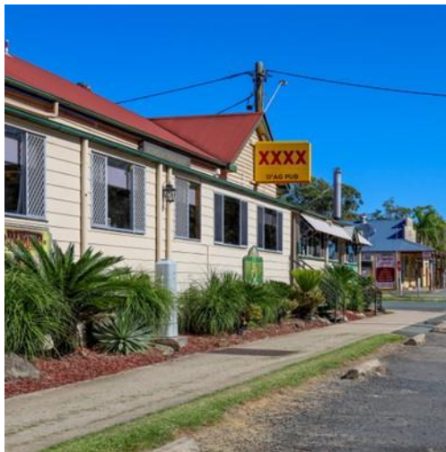
Dag Pub and Motel illustrates traditional colours and materials with its timber weatherboards and corrugated iron roof
