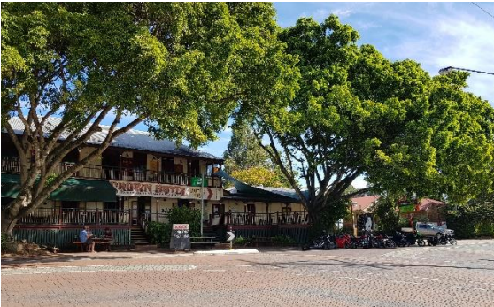
Crown Hotel provides a good example of the distinct character of the town and is located on a key site.
