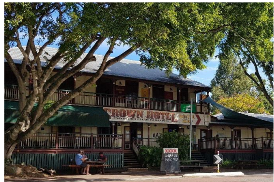
The Crown Hotel is in a prominent location 'overlooking' the town at the top of the hill. The large trees frame the traditional building.
