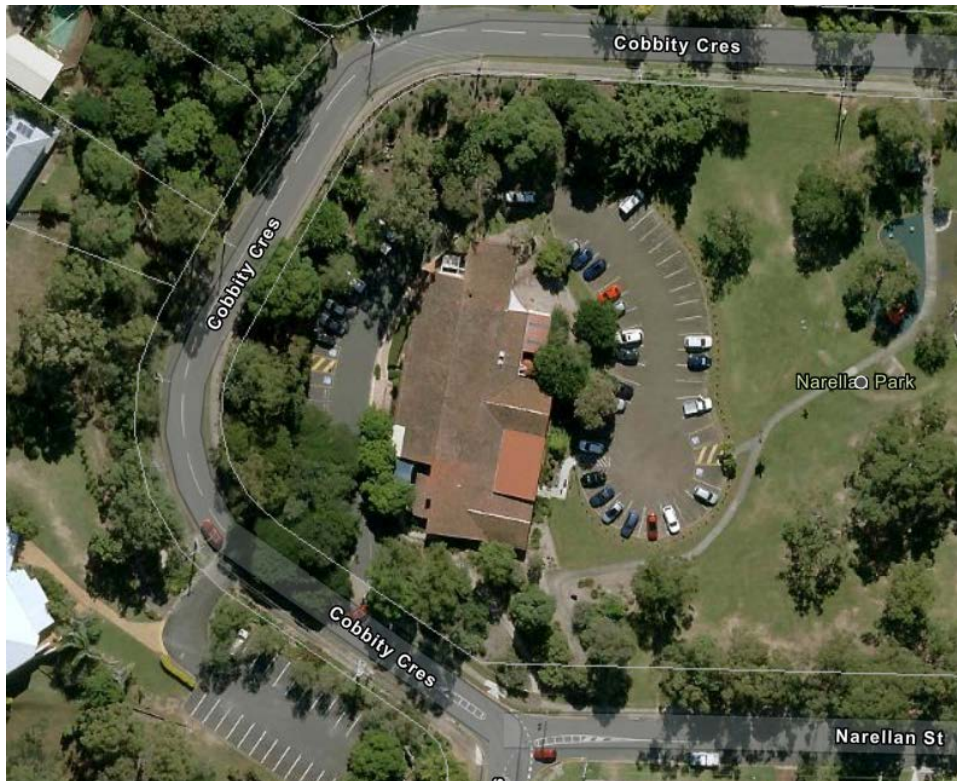
Figure 1: Location of works - Arana Hills Library
