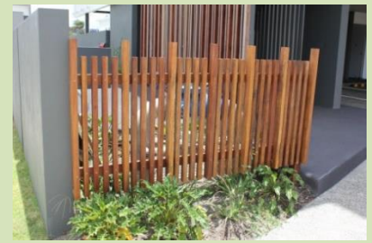
(Maroochydore) Semitransparent screening combined with landscaping can reduce the visual dominance of utilities while maintaining their visibility.
