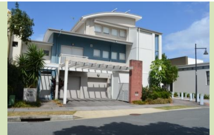
(Varsity Lakes) Dual occupancy on a corner
