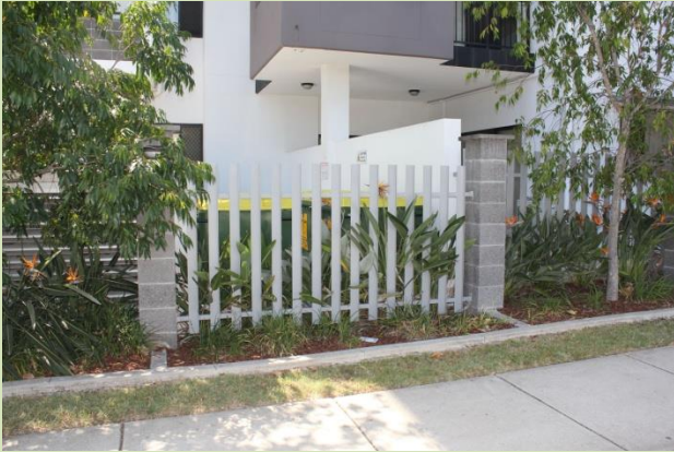
(Chermerside) Bin storage areas are to be screened and aesthetically treated to not be overbearing or visually dominate the streetscape.
