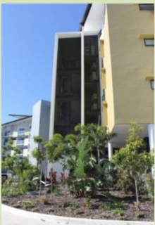
(Kawana) Screening of stairwells, and air conditioning units whilst maintaining ventilation.
