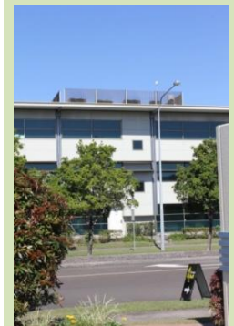
(Kawana) Screening of roof top structures needs to be considered.
