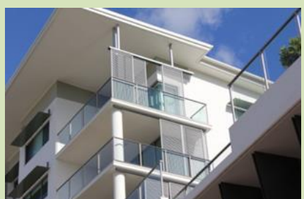
(Maroochydore) design solutions such as louvered screens with specific views, operable or fixed vertical louvres or planter boxes along the edge of balconies should be utilised to limit sight lines. Obscure glazing is the least desirable screening method for apartments.
