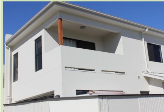
(Maroochydore) Solid balustrading can provide privacy to balconies whilst also facilitating surveillance.
