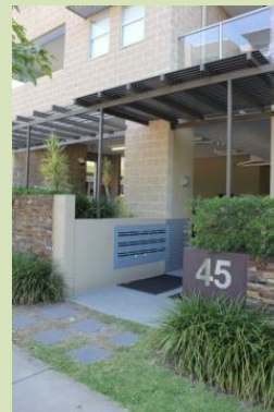
(Chermside) Mail boxes should be protected from weather, located close to the building entry so as to not create conflict between pedestrians and vehicles. Mail boxes can achieve good streetscape outcomes where they strengthen the sense of address for the building and activate the street frontage.
