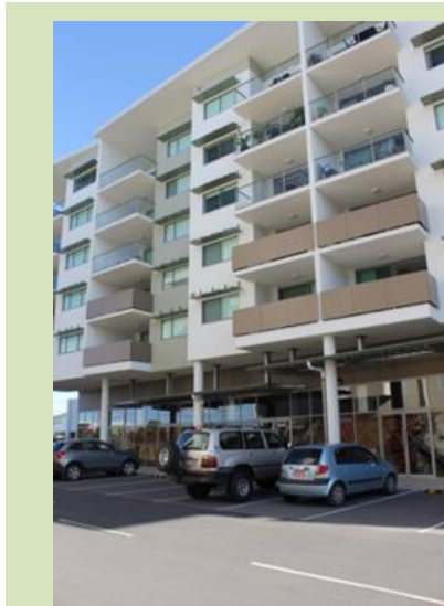
(Maroochydore) Solid balustrading for lower level apartments increases privacy while maintaining casual surveillance.
