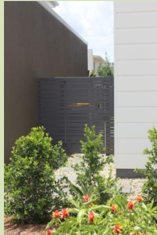
(Maroochydore) High fencing in line with the main building line with a gate can provide both screening for bin storage areas and ensure convenient access to collection point.
