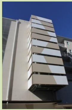
(Maroochydore) Screening of air conditioning units can add visual interest to the building.
