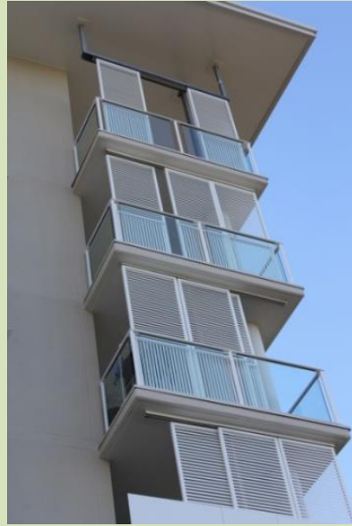
(Maroochydore) Sun screens, pergolas, shutters and operable walls should be utilised to control sunlight and wind.
