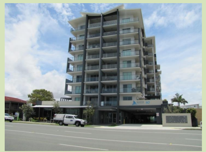
(Clontarf - Front on view to see screening treatments in effect) Mail collection, landscaping and an architectural feature forming part of the building all work together in this example to reduce the visual dominance of ground floor car parking areas.
