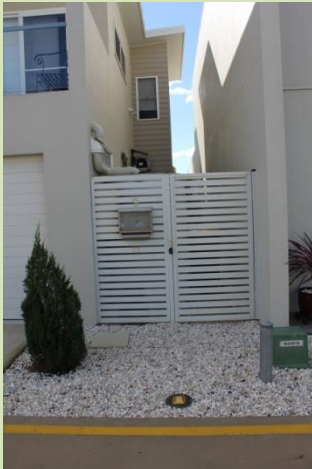
(Maroochydore) High fencing in line with the main building line with a gate can provide both screening for bin storage areas and ensure convenient access to collection point.
