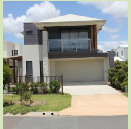
(Maroochydore) • Garages should be setback at least 1m behind the main building line. • Car ports and domestic outbuildings should not be located within the front setback. • For 2 storey buildings the garage should be recessed back from the second storey.
