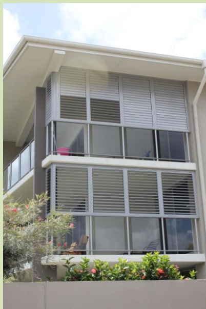
(Cotton Tree) Breezes are blocked when screens are not carefully designed. Adjustable screens can block sun when needed and provide privacy for both occupants and neighbours.
