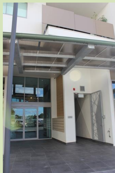
(Maroochydore) Separate entrance for residential uses should be provided in mixed use buildings.
