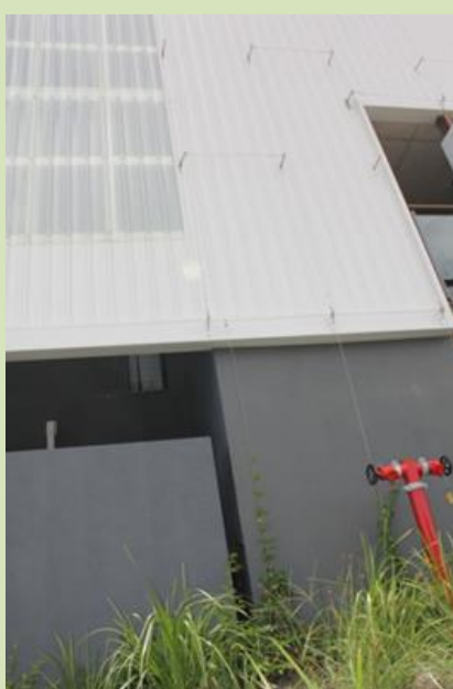
(Maroochydore) Greening streetscape e.g Green walls with the help of climbing species
