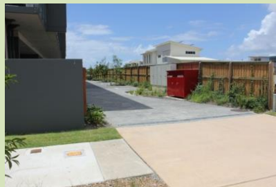
(Maroochydore) Services such as fire hydrants and electrical transformers should not be visually prominent at the streetscape. Screening and landscaping should be utilised to reduce the visual dominance utility areas have on the streetscape and adjoining sites.
