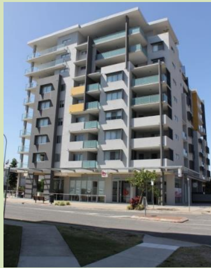
(Chermside) High buildings provide vertical articulation through a distinct top, middle and base section.
