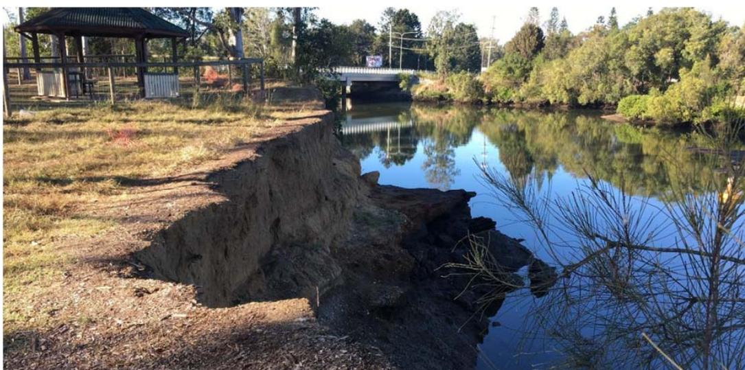
*Figure 23 - Erosion Scarp at Wylie Park (prior to Bank Stabilisation works) on North Pine River, just upstream of the Gympie Rd Bridge*
