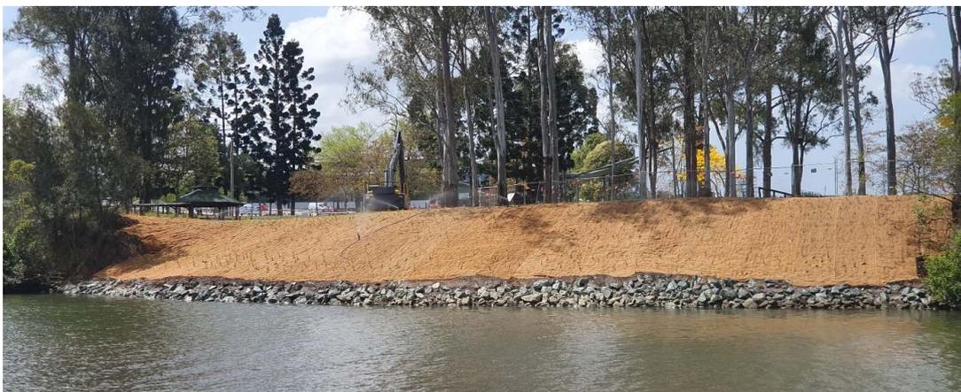
Figure 26 - After completion of bank stabilisation works
