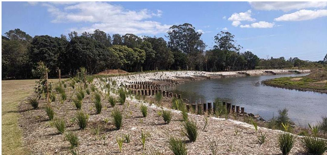
Figure 1 - Example of recently constructed bank stabilisation works at Pine Rivers Park, South Pine River
