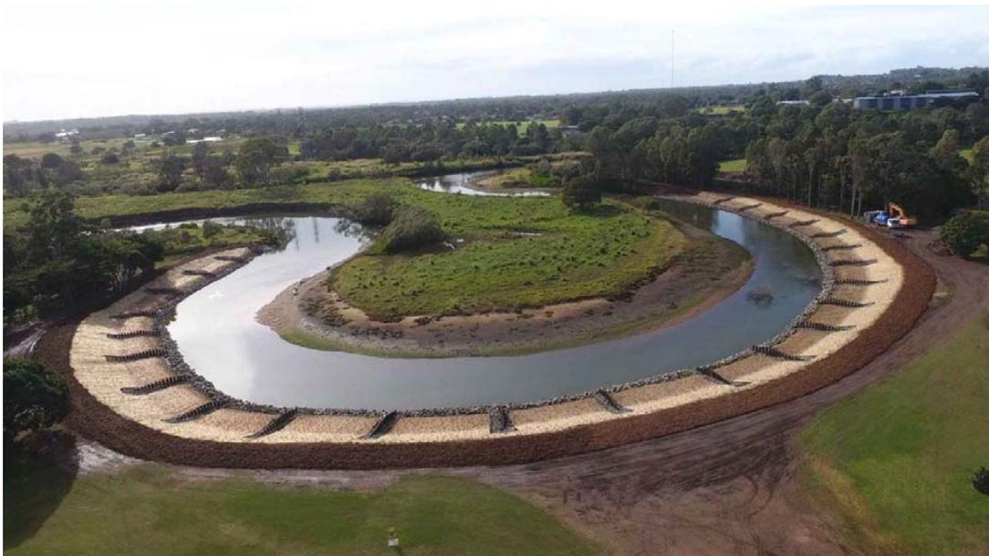
*Figure 15 - Aerial view of completed bank stabilisation works at Pine Rivers Park, South Pine River*
